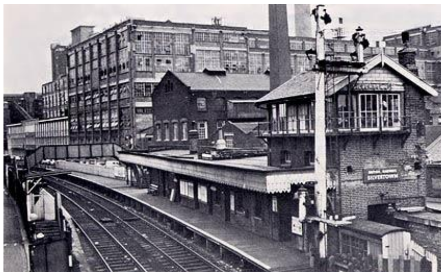
9 Silvertown Railway Station 1965
