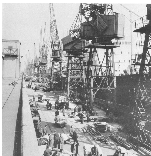
3 Albert Dock quayside, a busy scene in the late 1950s
