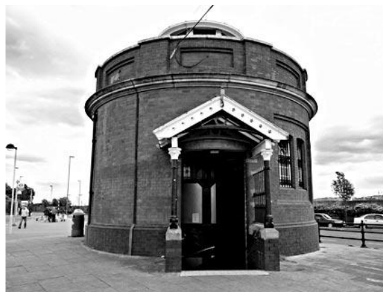
7 Foot tunnel entrance at Woolwich
