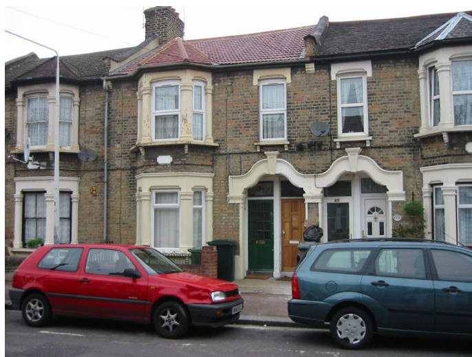
27 No. 39 Ling Road 2006 (new brown wood door)
